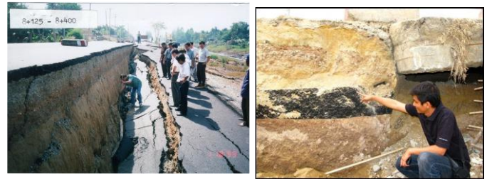
Fig.3 Problems of slope failure and differential settlement in Soft Bangkok Clay
